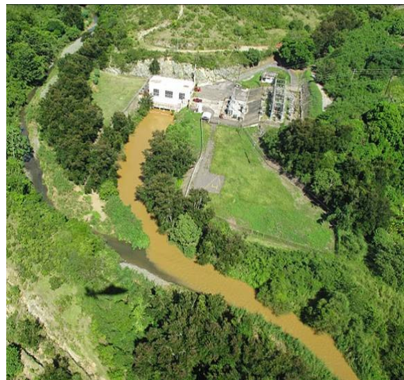
Figure 2: The pumphouse into Lago Loco reservoir from Lago Lucchetti demonstrating interbasin transfer of sediment.
